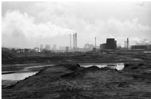
Lignite power plant in Espenhain.
